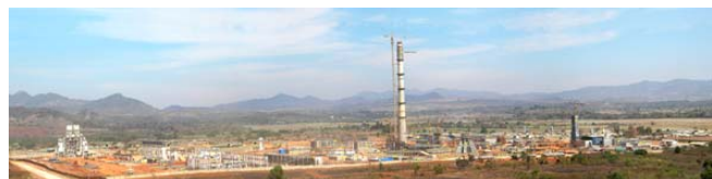
Fig. 3 General view on the site of the Romelt plant in Myanmar
